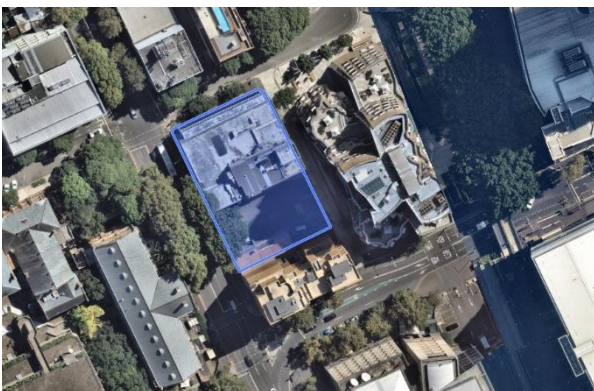
Figure 6: aerial, 622-644A Harris Street
